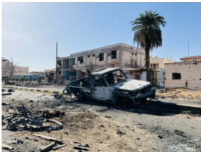
Figure 4: The damage to the Al-Shaab Teaching Hospital in Khartoum (Human Rights Watch, 2025)
